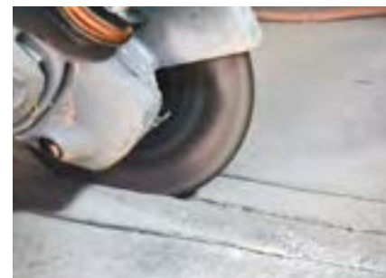
Creation of traces on reinforced concrete.
