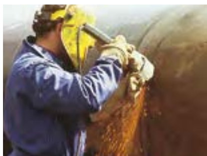
Creation of traces on reinforced concrete.
